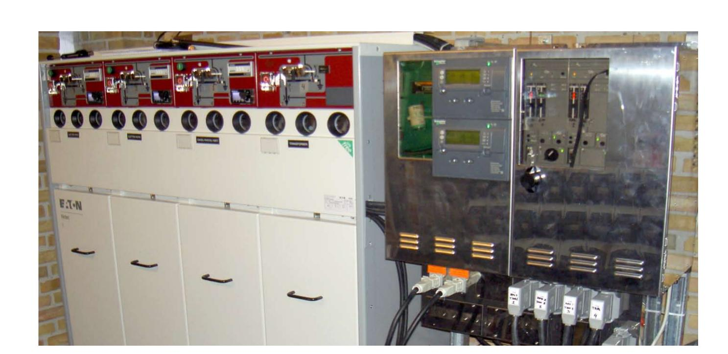
2 SACSe substations divides the feeder into 4 fault sections.
